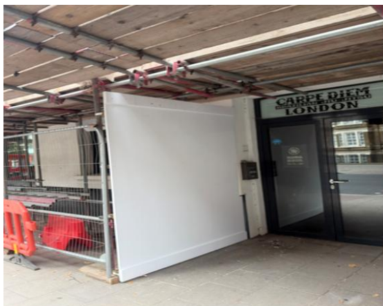
A photo of the protective gantry and hoarding surrounding the building entrance, ensuring residents can enter and exit safely while construction works take place above.
