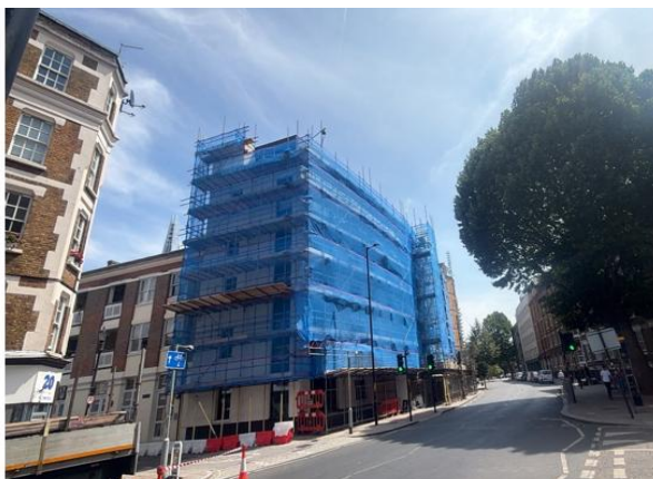
A photo of the Scaffold erection complete
