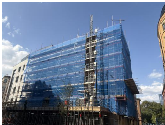
A photo of the Scaffold erection complete
